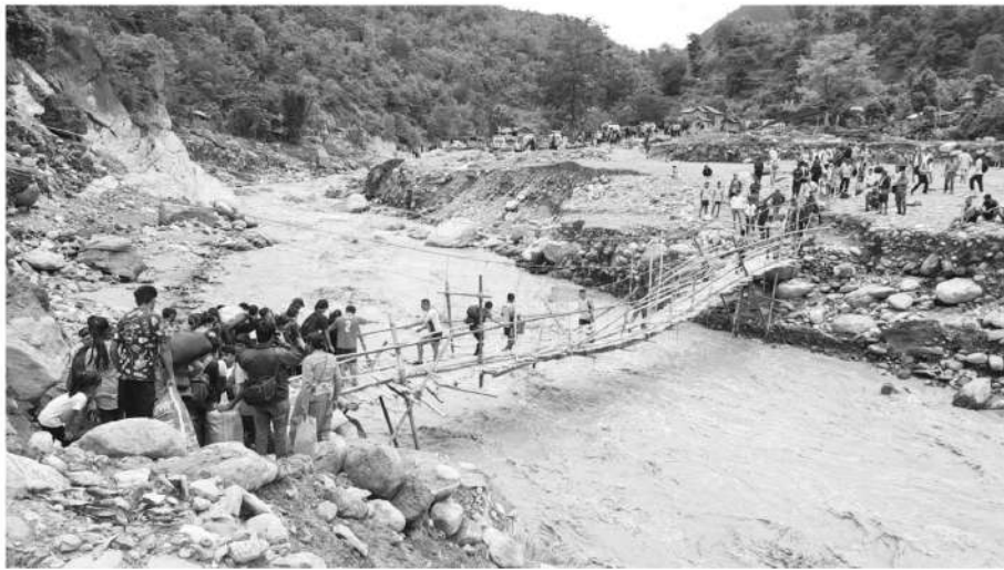
RISKY JOURNEY: People crossing a bamboo made temporary bridge over Heva Khola River in Panchthar as the concrete bridge over the river was swept away by the swollen river due to monsoon rains.
